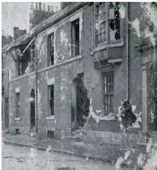
Damage to Moor Street © Hartlepool Borough Council.
