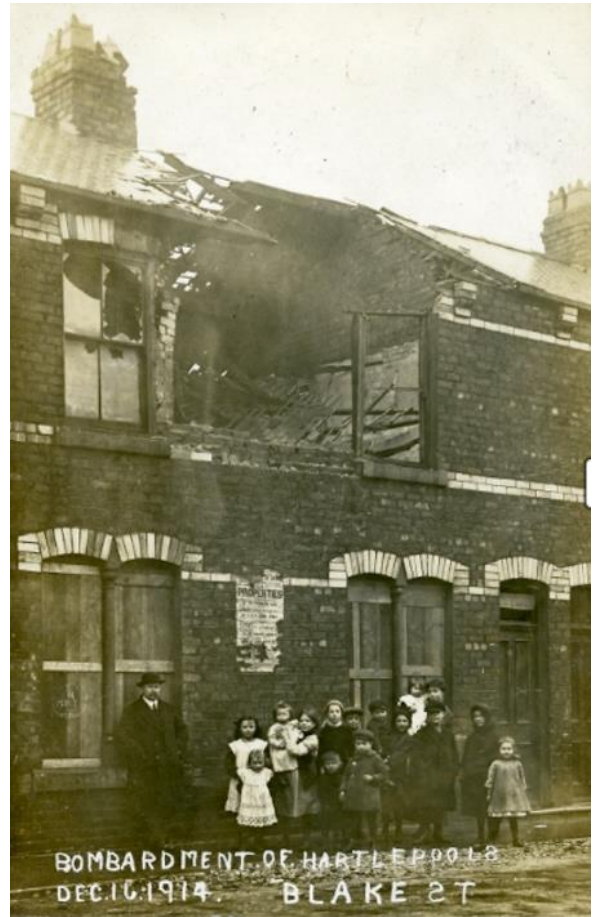
Damage to a house in Blake Street © Hartlepool Borough Council.
