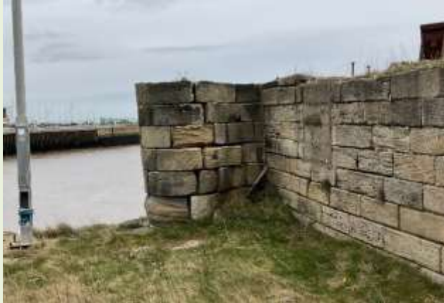
Condition prior to repairs
