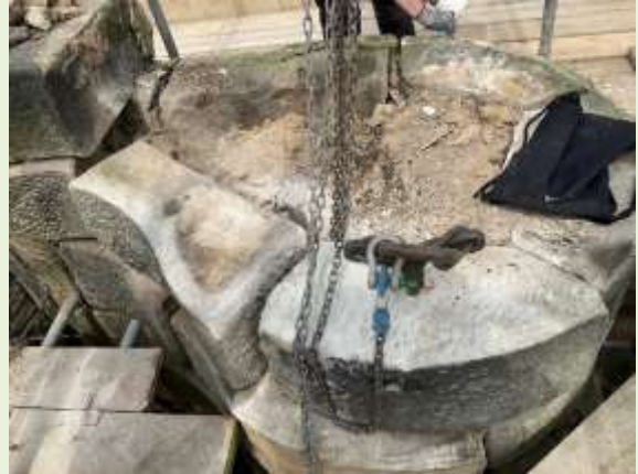
Lifting and removal of stones for re-bedding and repointing.
