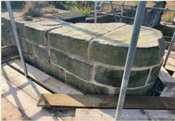
Completed repairs prior to scaffolding being removed
