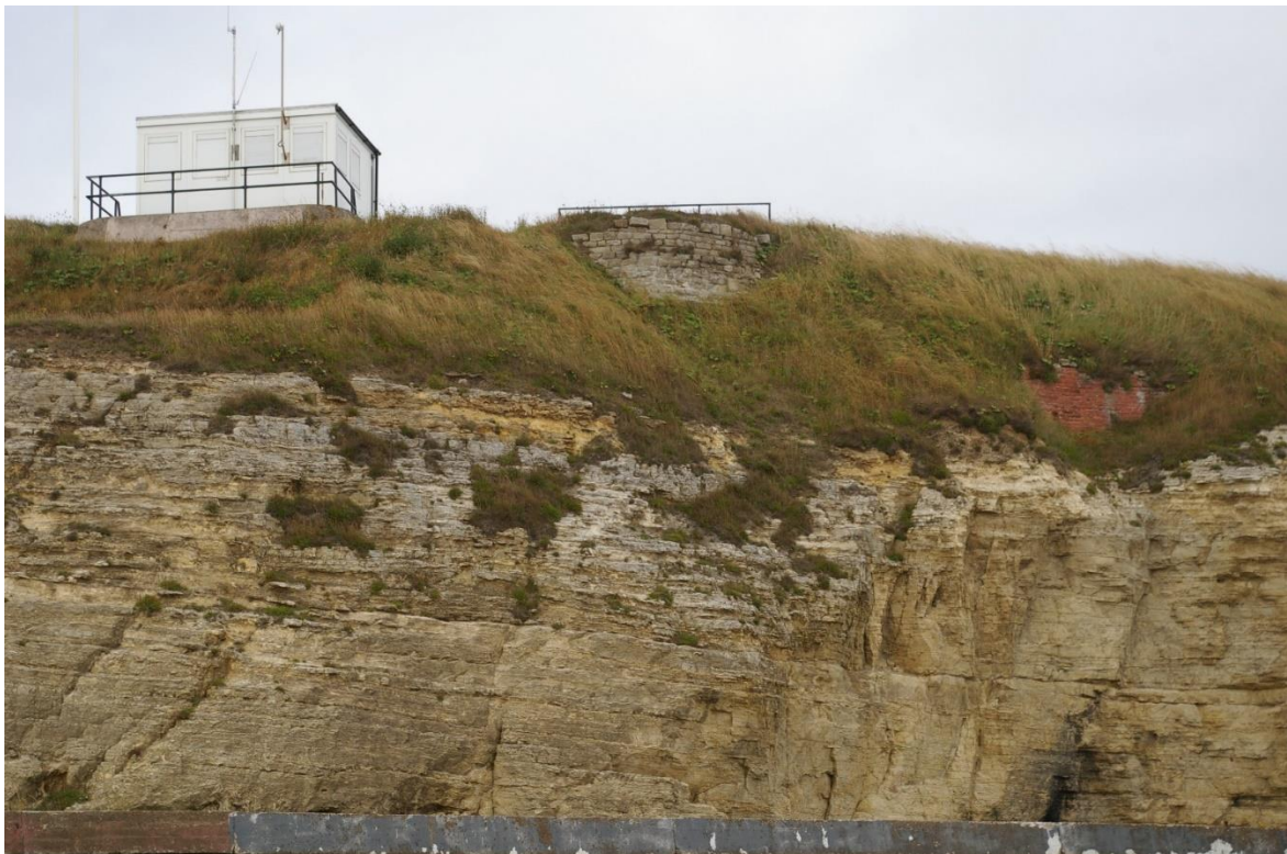
Figure 26: Remains of pre-First World War gun battery in east facing cliff face
